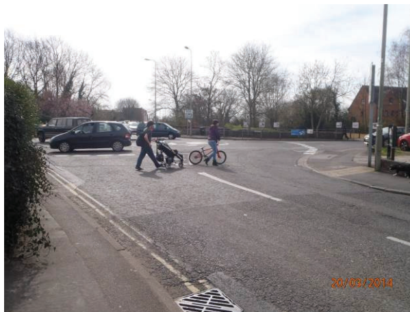
Photograph 1 - Three pedestrians, one of which was pushing a pushchair were observed crossing Spring Road via the existing uncontrolled crossing facility.
